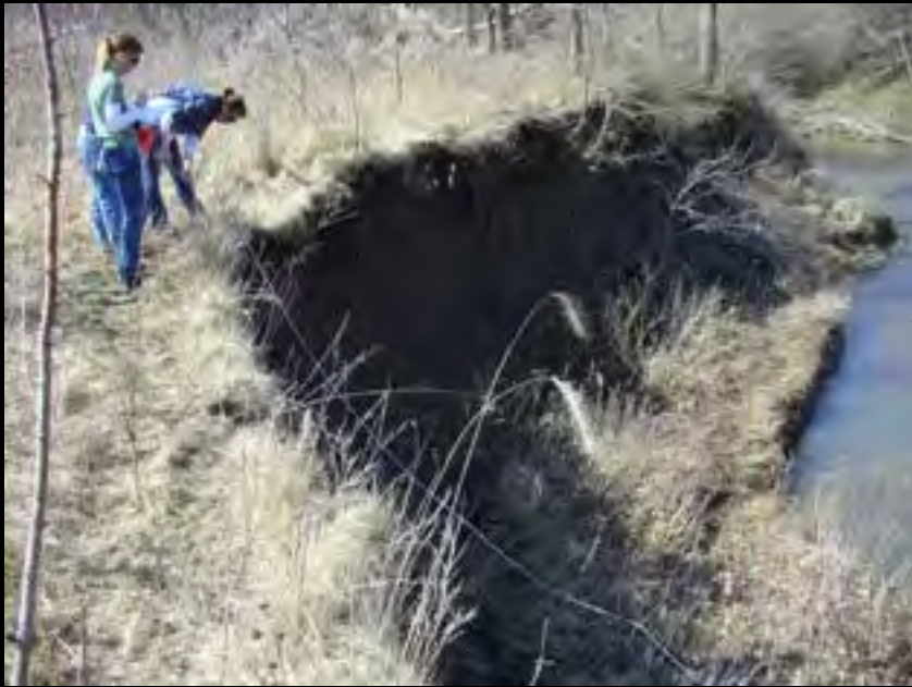
Kansas Water Office Photo ( kwo.org )
